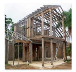
This oversight can lead to significant risks, as prolonged exposure to the elements will compromise the integrity of the timber structure. The timber components are likely to warp, split, and suffer from fungal damage. Nail plates will show signs of surface corrosion with teeth backing out losing its grip. Additionally, the trusses will lose their camber and experience increased creep deflection under service load.
