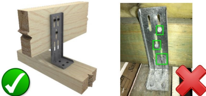
Fig. 6 - Nails should not be overdriven or fixed at the bottom slots
