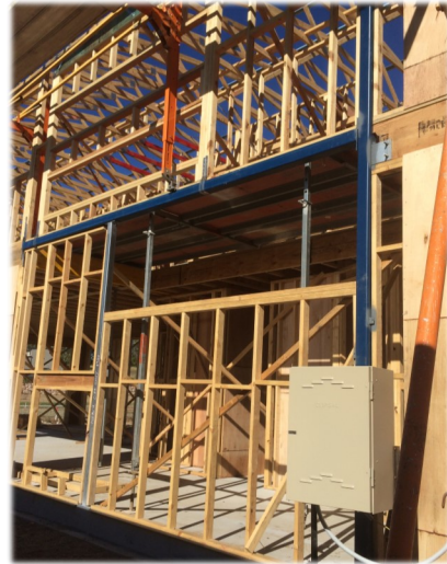
Images above and below show a typical 90x90 SHS steel wind beam and column that were installed to keep the wind beam size down when timber was not adequate.
