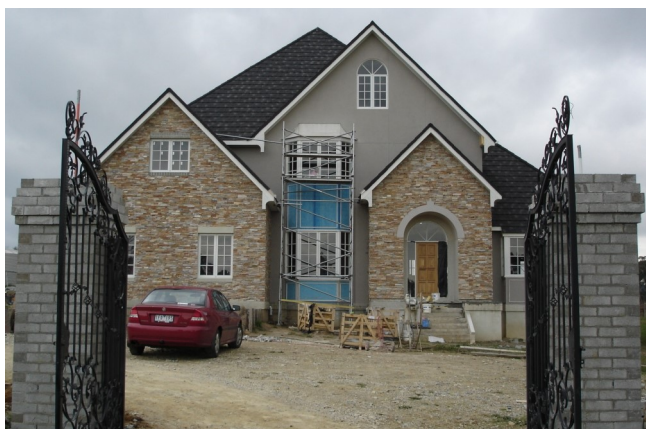
Fig. 1 - Two storey dwelling with 40 deg. roof pitch
