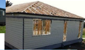
Day 4 & 5- Roof trusses, fascia & gutter
