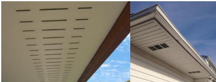
Figure 3 – Continuous eave vent (Left) and spaced eave vent (Right)
