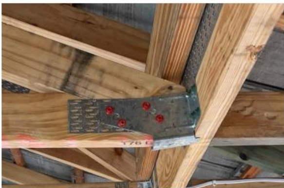
Figure 4. Girder bottom chord rotation on site
