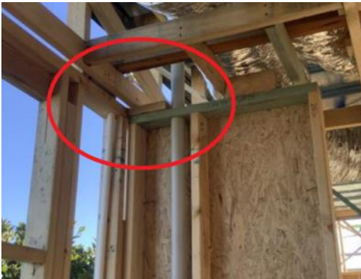
Photo 1 - Example of plumbing pipes through wall plates
