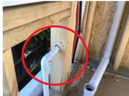
Photo 2 - Example of plumbing pipe through jamb stud
