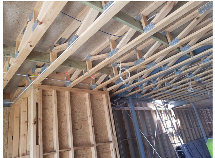
Strongbacks help to reduce bounciness
