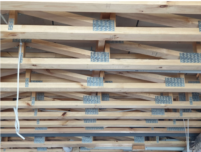
Strongbacks help to reduce bounciness
