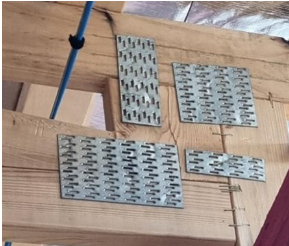
Figure1 – Splitting in short swan timber member after pressing
